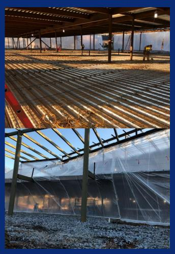
Main and 2<sup>nd</sup> level provided with temp heat and enclosure to facilitate 2<sup>nd</sup> level concrete pour
